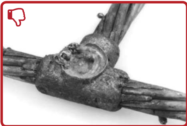
Light carbon traces on cable and connection are evidence of oil on cable strands. Oily cables must be cleaned with safety solvent.
