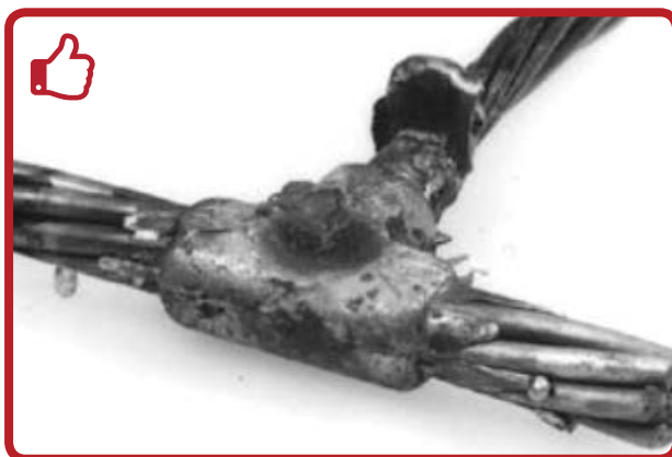
A worn or incorrect mold was used, allowing leakage around conductor. The fill in this connection is sufficient to allow it as acceptable. Attention to mold is required prior to making next connection.
