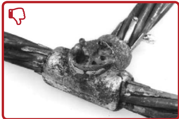
Heavy carbon coating on cable and connection is evidence of large amounts of oil or grease on cable. Cable must be cleaned with safety solvent.
