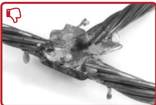
Fill too low. Weld cavity was not filled over cable strands. "Fins" indicate that the mold was not closed tightly due to incorrect mold, incorrectly adjusted handle clamp, or presence of foreign material in mold parting line. Before making the next connection, check the mold for each of the above.
