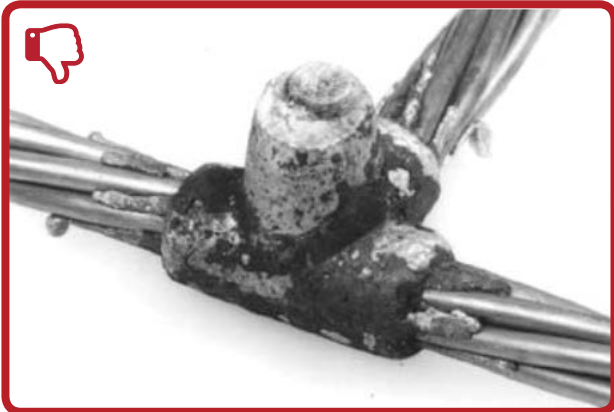
Extreme amounts of slag on surface are caused by welding material leaking past disk or complete lack of disk. Inspect the condition of mold disk seat and check disk positioning prior to making the next connection.
